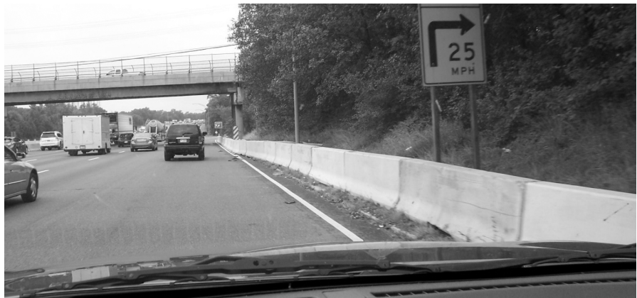
Figure 3-9: A Jersey barrier
